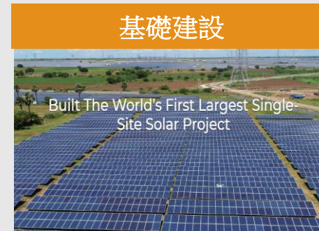
Greenko Solar (India)
